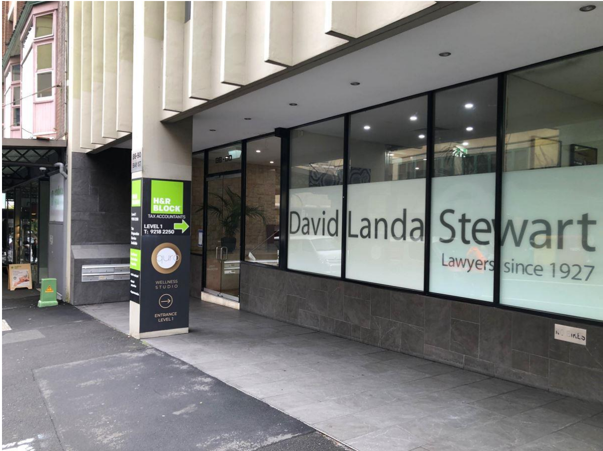
Figure 4: Site viewed from Bay Street looking north
