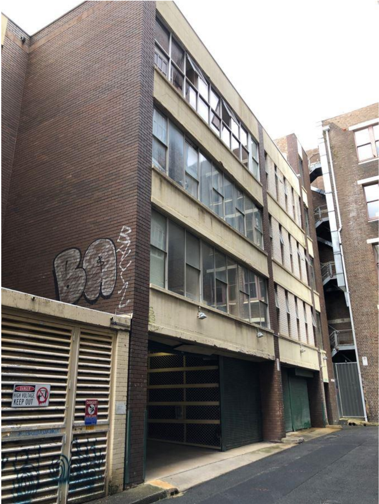
Figure 7: Site viewed from St Barnabas Street looking west
