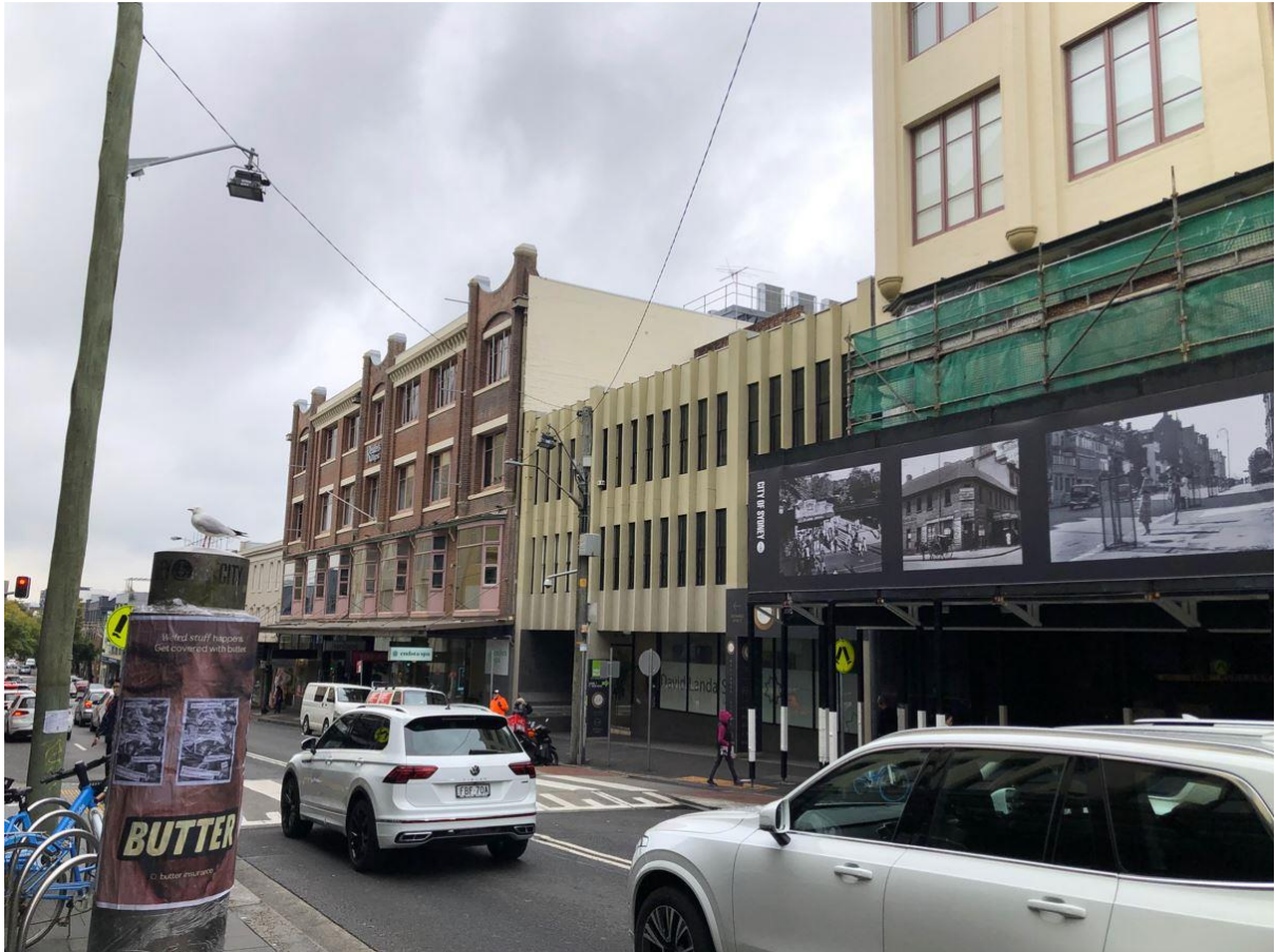
Figure 5: Site viewed from Bay Street looking north
